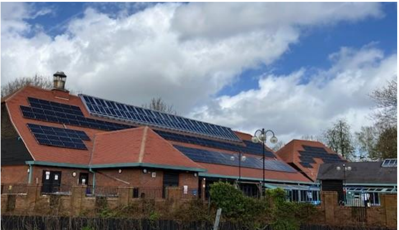
Solar panels on the roof of Tonbridge Swimming Pool
